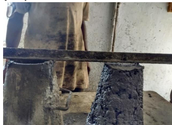
Slump cone test
